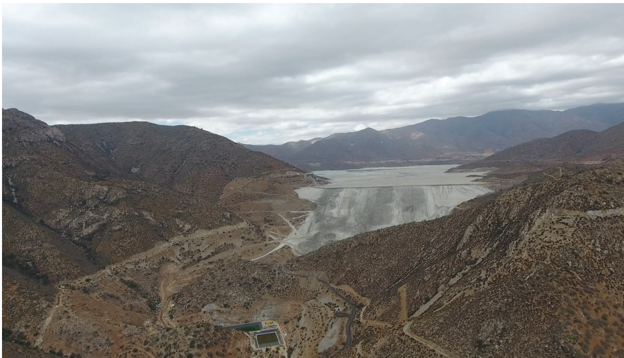
Figure 3. El Mauro tailings dam. Drone footage from fieldwork conducted in March 2021.
