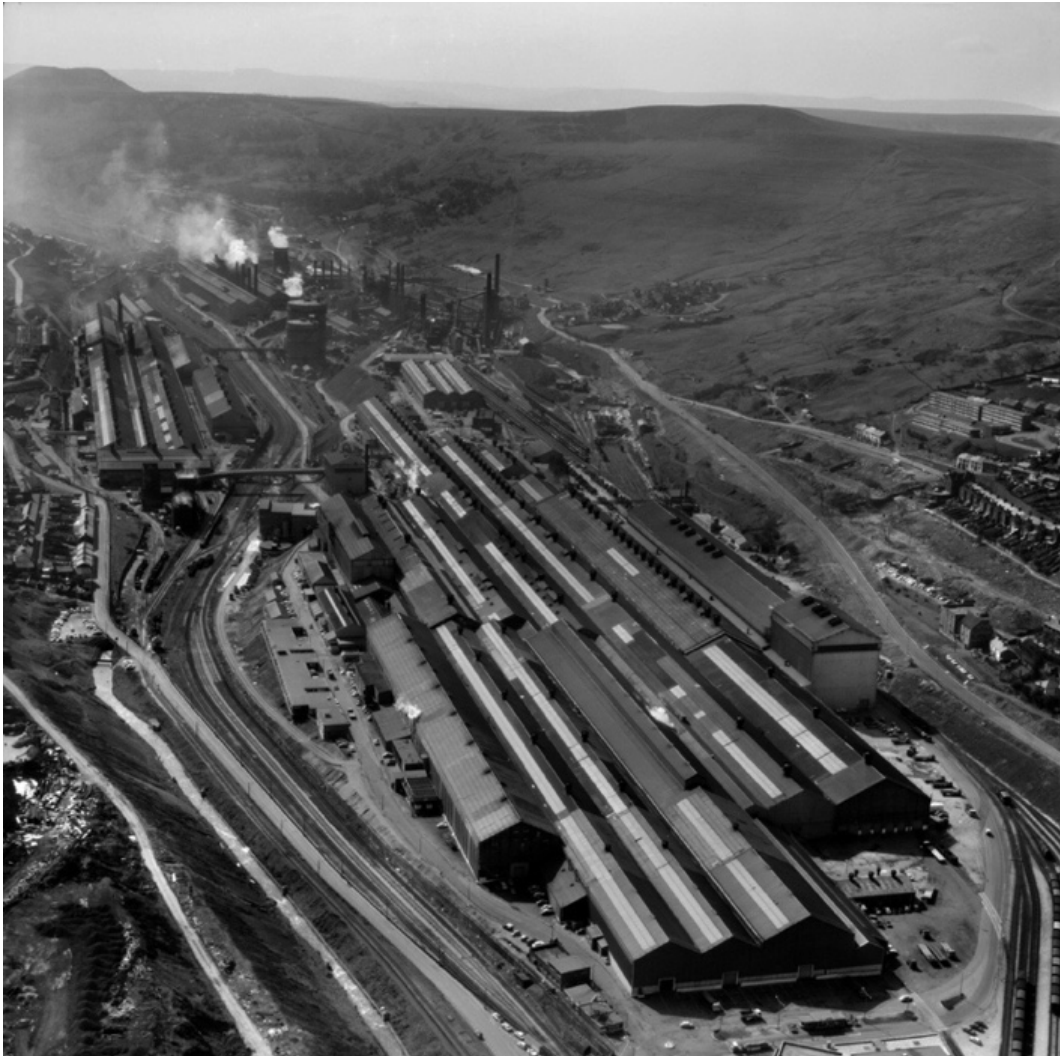
Fig. 4. Black and White oblique aerial photograph showing the steelworks at Ebbw Vale, Aerofilms Collection (Monmouthshire: 1972). Looking south from Ebbw Vale town. At the top of the picture are the blast furnaces and later the location of Garden Festival Wales. © Crown copyright and is reproduced with the permission of the RCAHMW.
