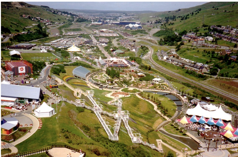
Fig. 7. Anne Marie-Lewis, View from the Sky Shuttle, Garden Festival Wales (1992). Looking north across the festival site (to the middle ground is the former location of the steelworks blast furnaces) to Ebbw Vale town. At the top of the picture, part of Ebbw Vale steelworks which was still in production at the time. © Anne Marie-Lewis.
