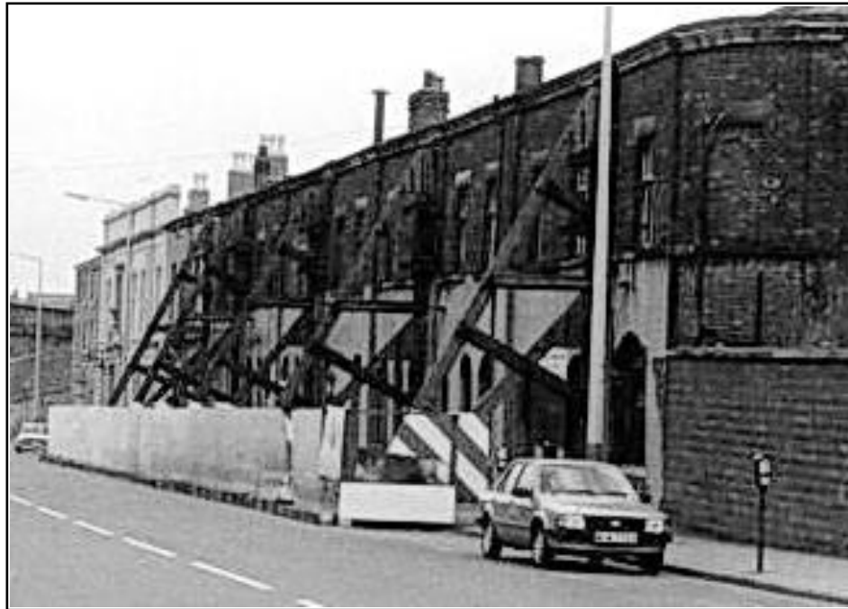
Figure 5.2 The soot blackened Liverpool Road Station supported by massive wooden shoring (1978) (MLIC)
