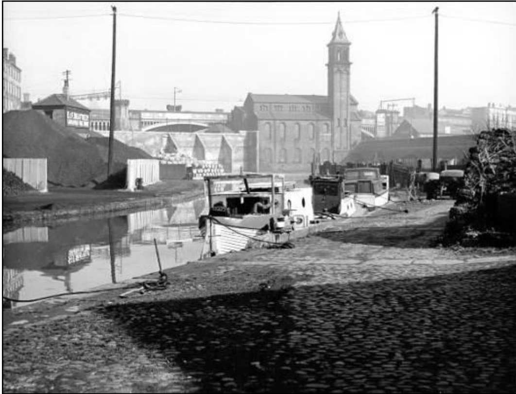
Figure 6.9 1960s Industrial canalscape photograph: Castle Quay and Coal Wharf with the site of Grocers Warehouse in the background behind the coal (source MLIC)
