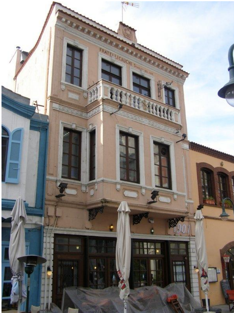
Fig. 3.3.xvii Cauchi Bros building on Katouni Street
