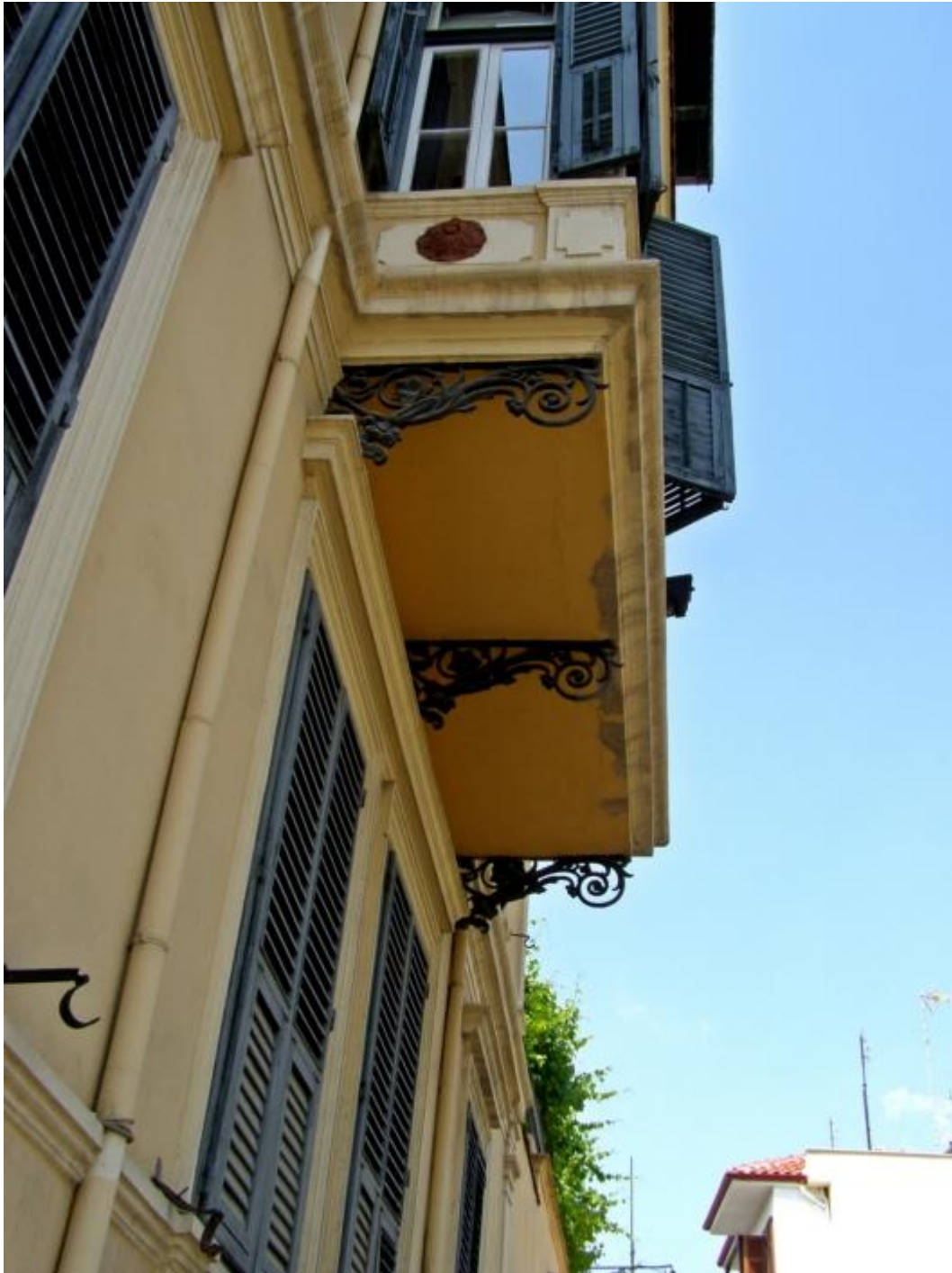
Fig. 3.3.88 The brackets of the above building
