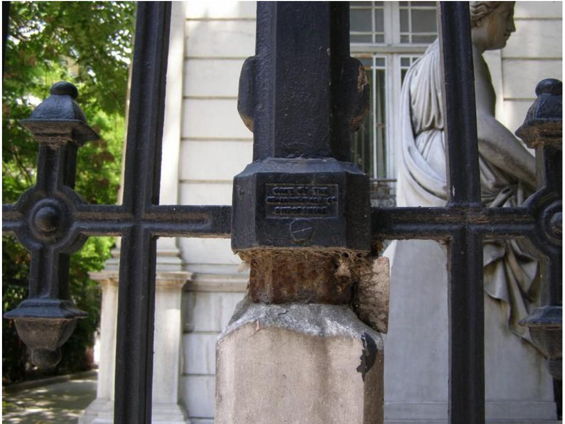
Fig. 3.3.43 Detail on the gate railings of the Ottoman Bank
