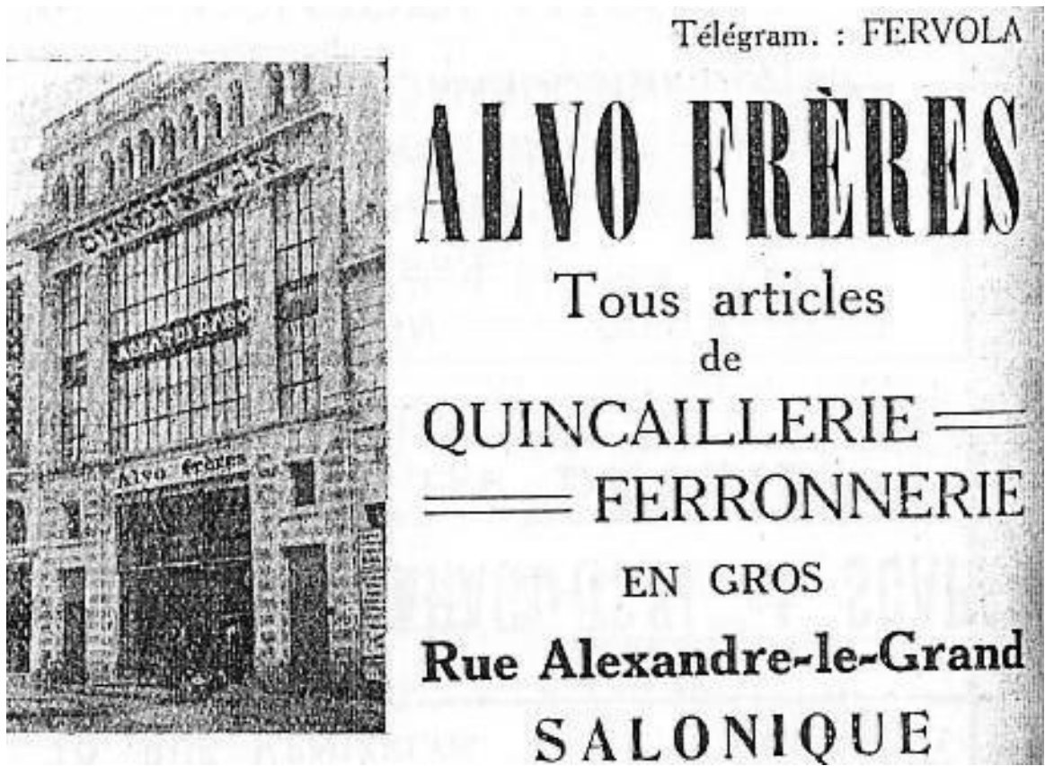
Fig. 2.3 The Alvo Brothers ironwork shops in Thessaloniki (early 1920s)
