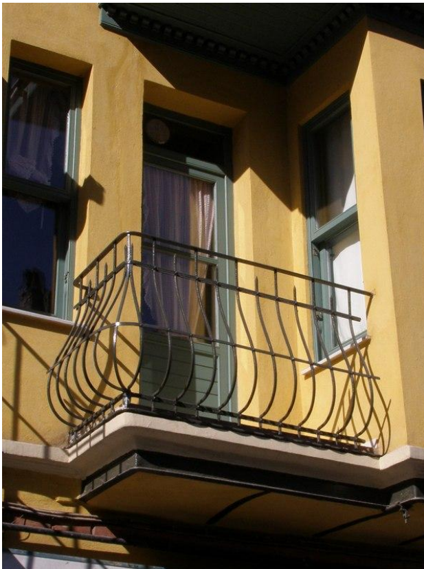
Fig. 3.2.84 Vodinya and Ayan Street
