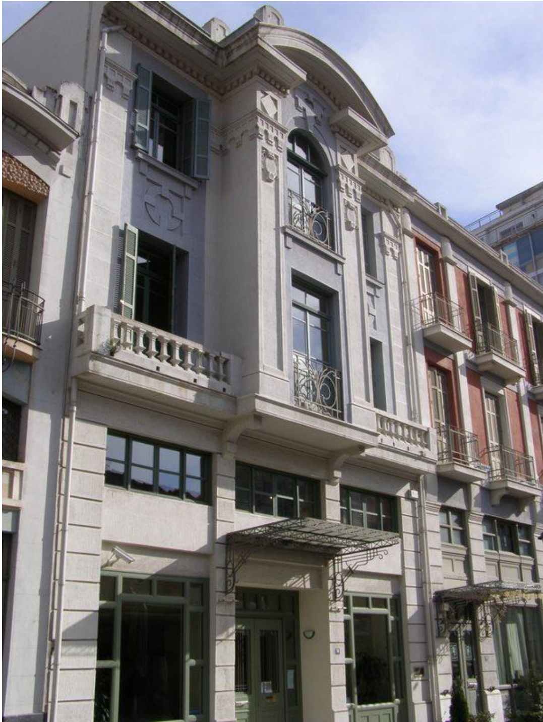
Fig. 3.3.xiv The building on Katouni Street 14
