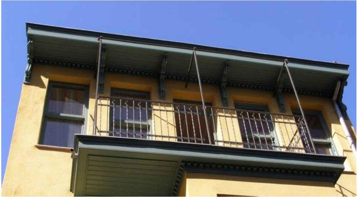
Fig 3.2.88 Vodinya and Ayan Street
