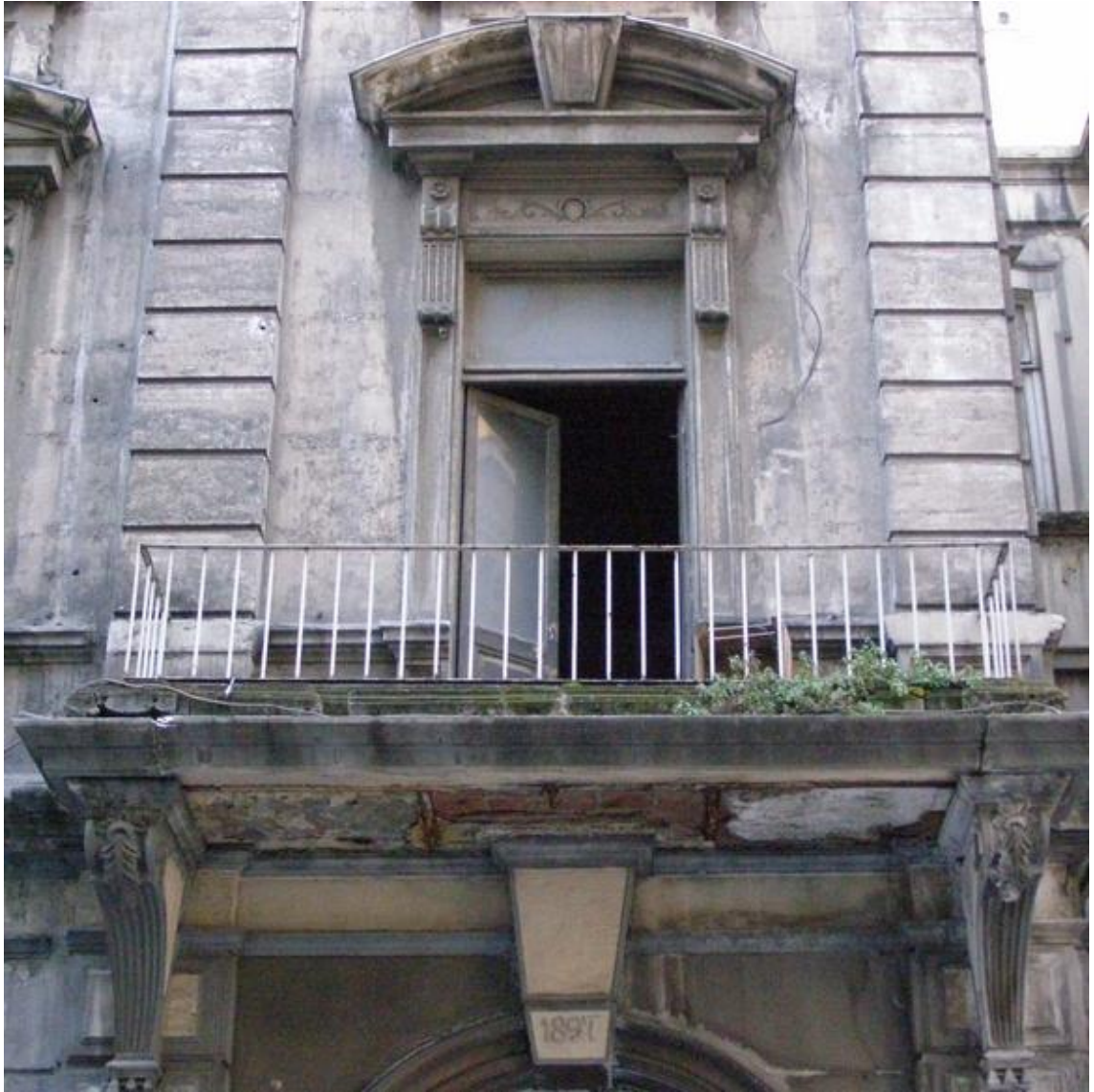
Fig. 3.2.70 Detail of the same building
