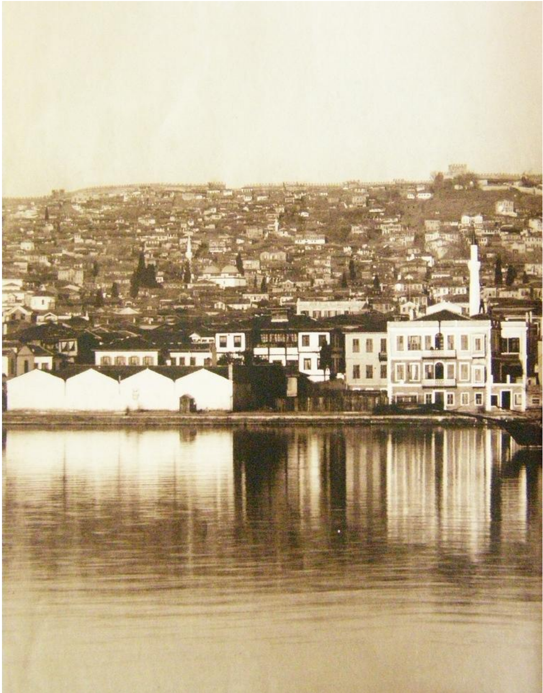
Fig. 3.3.viii The middle of the littoral front in early 1880s after the demolition of the sea walls
