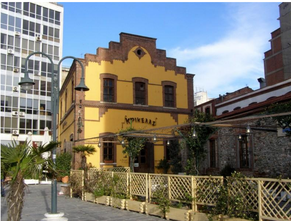
Fig. 3.3.xx Warehouse on Salaminos Street
