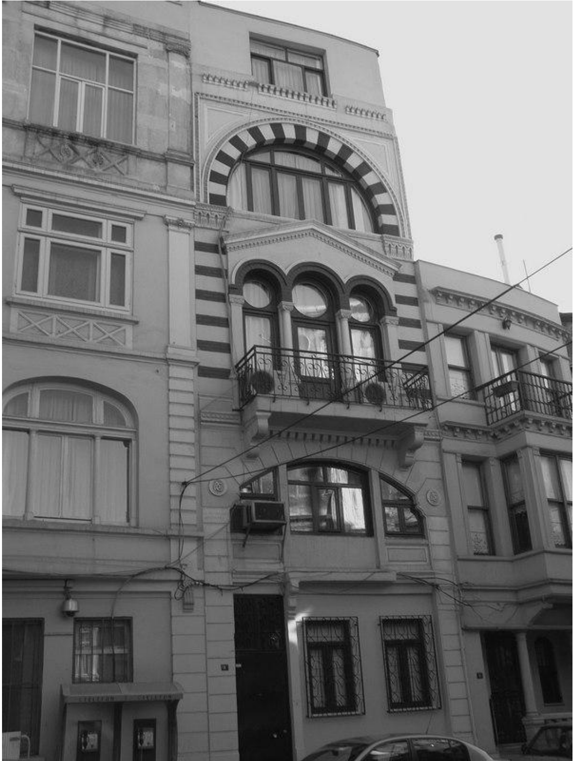
Fig. 3.2.90 At the vicinities of Marasleion, Vodinya Street 9.
