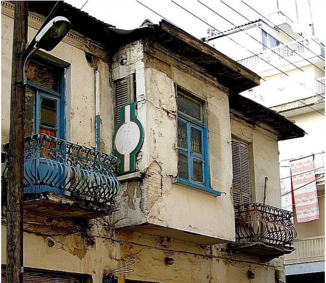
Figure 3.3.f. Detail of the same building
