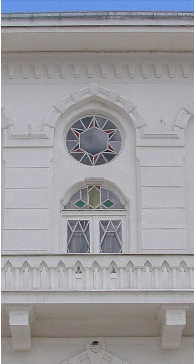
Fig 3.1.xxii Details of the southern façade
