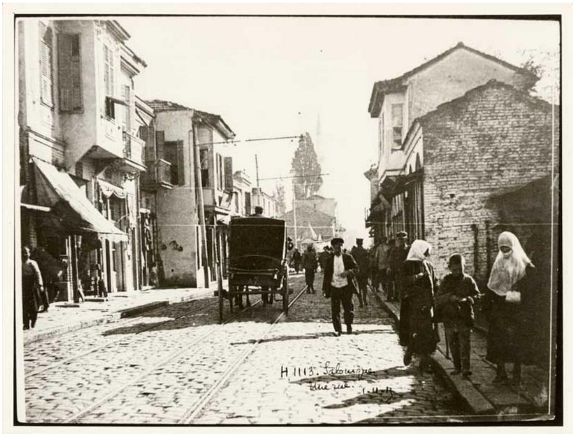
Fig. 3.3.15 An indefinable point on Egnatia Street
