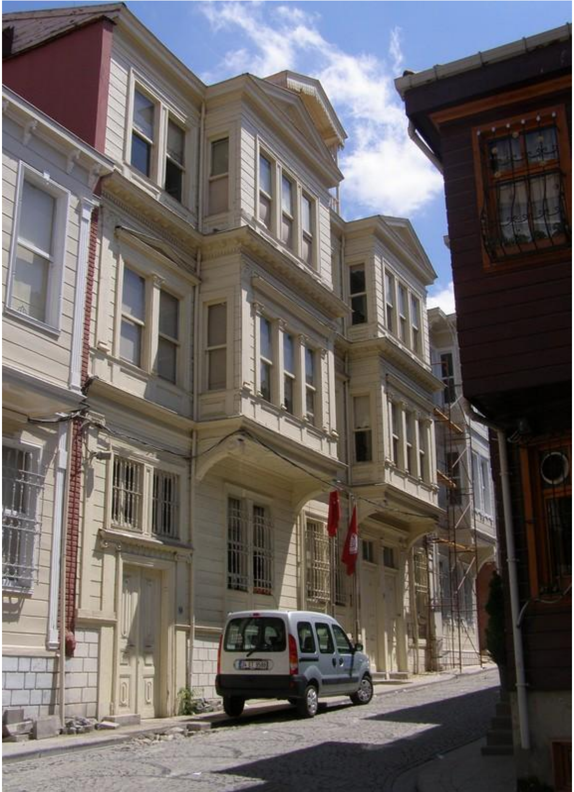
Fig. xlii The building of the center for restoration (KUDEB)
