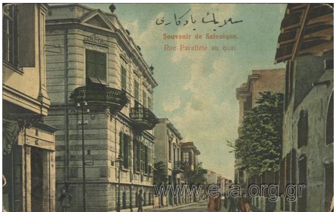
Fig. 3.3.3 View of a street parallel to the sea front
