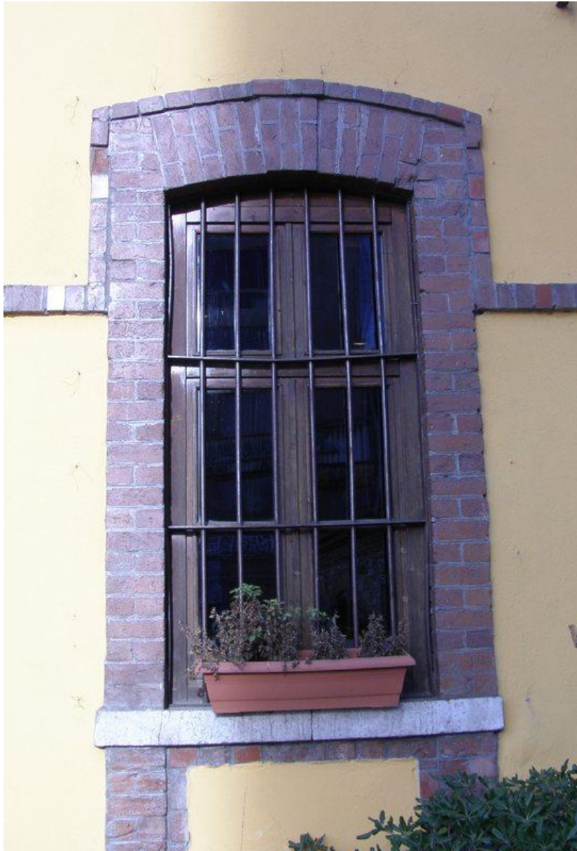
Fig. 3.3.xxi Window of the warehouse on Salaminos Street
