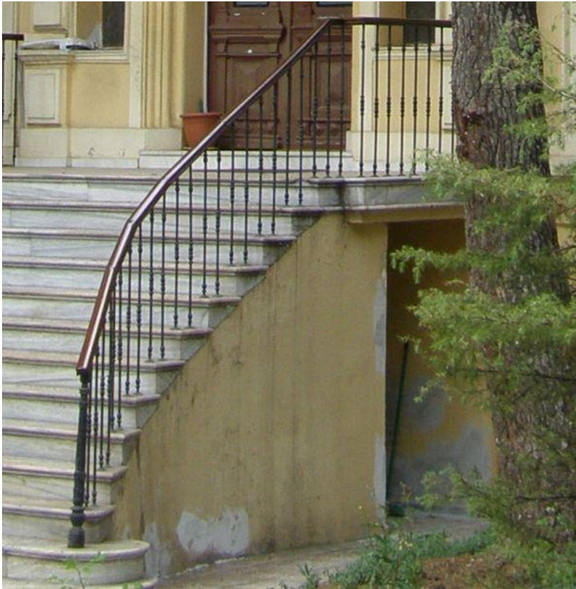
Fig. 3.3.51 The balustrade of the stairway
