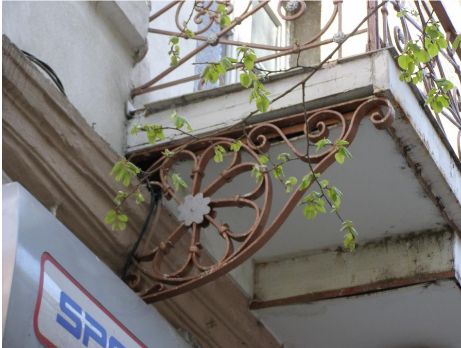
Fig. 6 One of the rare iron brackets in the area of the market
