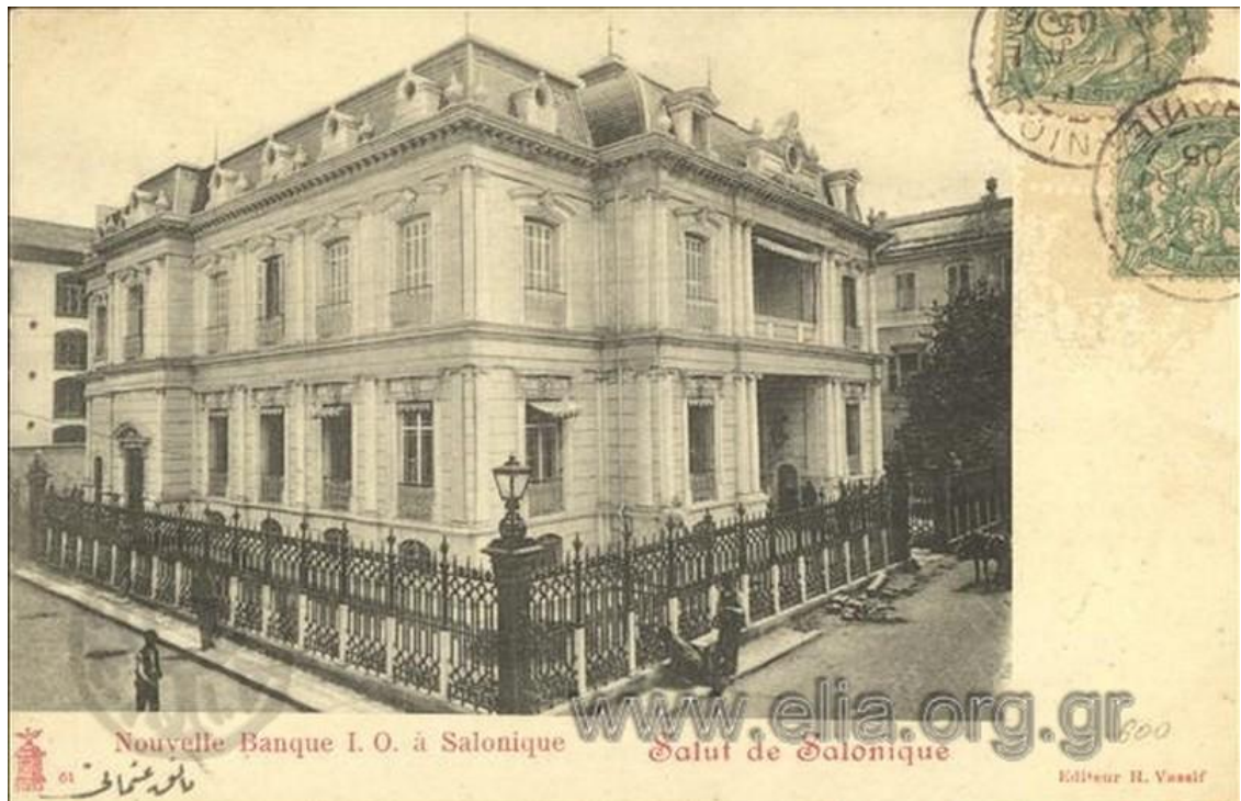
Fig. 3.3.42 The 'new' building of the Ottoman Bank
