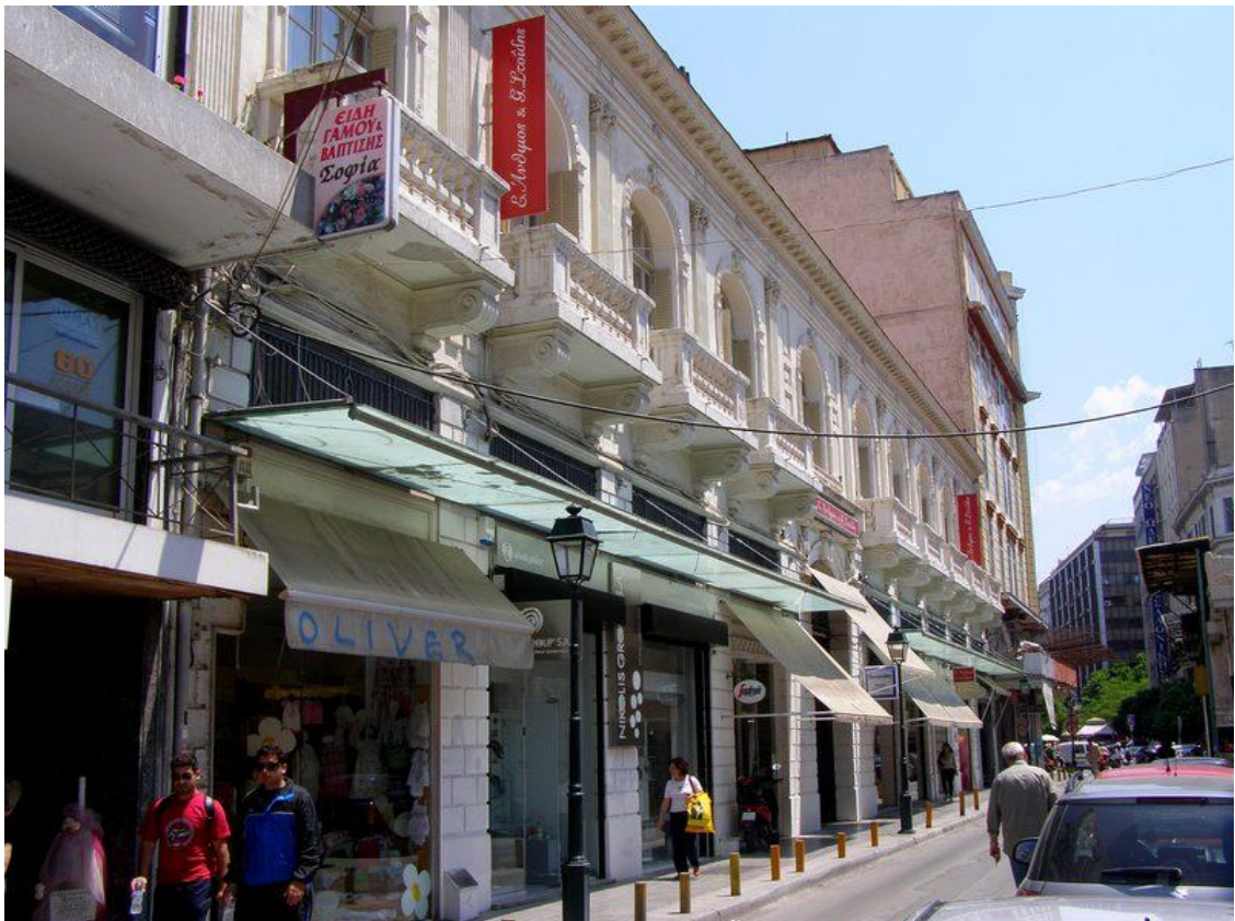
Figure 3.3.k. The Saoul Arcade; the façade on Vassileos Irakleiou Street
