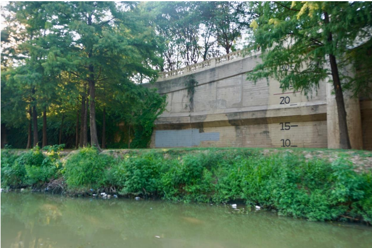
Fig. 32. Flood levels at the Buffalo Bayou, July 2019. During Hurricane Harvey, the Buffalo Bayou rose to a record 39 feet at the Shepherd Drive Bridge. (Image credit: Kate Pickering)
