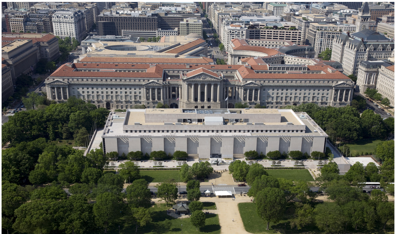
[Fig. 7: In the foreground, the building housing the current-day National Museum of American History, originally opened in 1964 as the Museum of History and Technology. The surrounding buildings are emblematic of the classical style common to many buildings located on and around the National Mall.]
