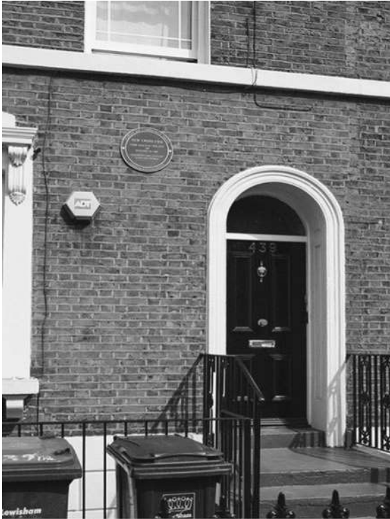
Fig. 3.8 439 New Cross Road
