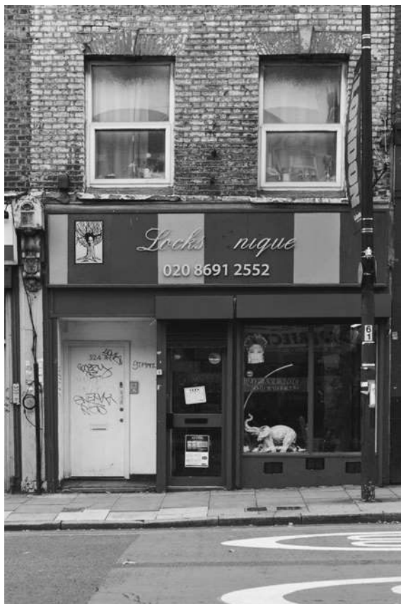
Fig. 3.6 324 New Cross Road
