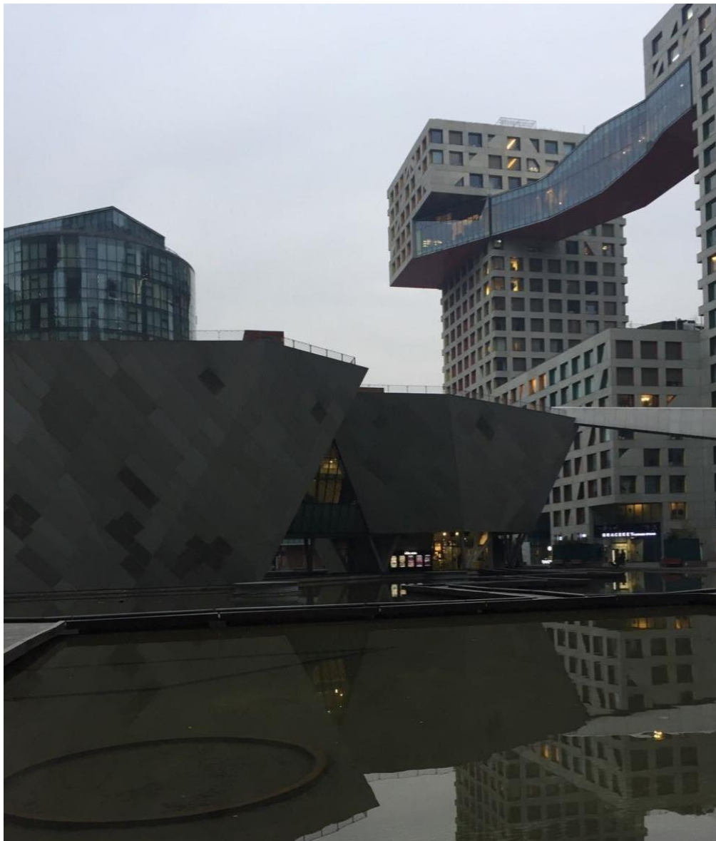
Figure 18. Modernist architectural style of the BC-MOMA.
