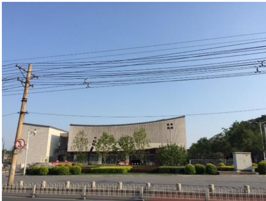
Figure 7 Tianqiao Performing Arts Area, Beijing © Xiao Lu
