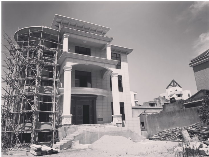
Figure 23. A house under construction in Fuqing.
