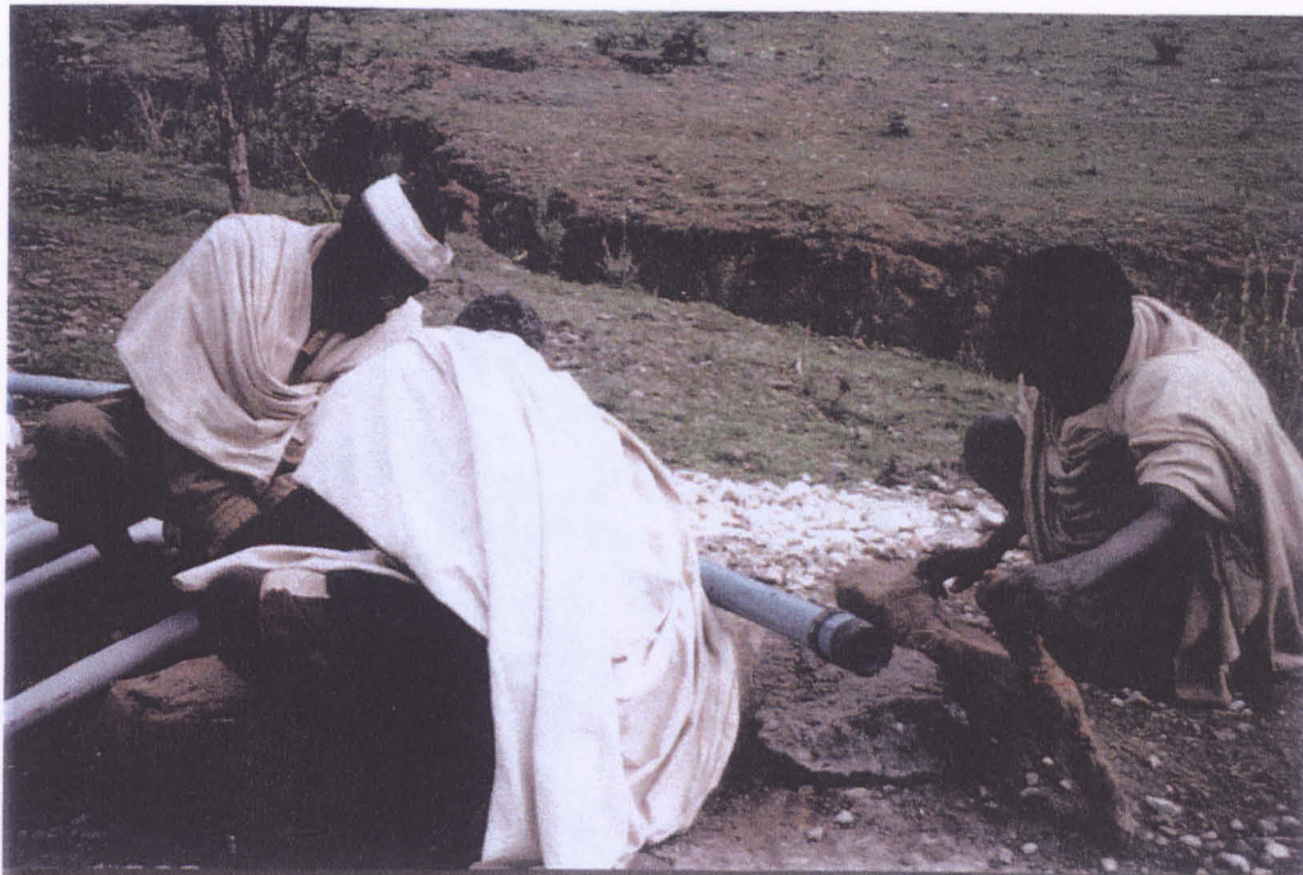
Figure 6.5 Men put hand pump parts together at Kollo Tembien
