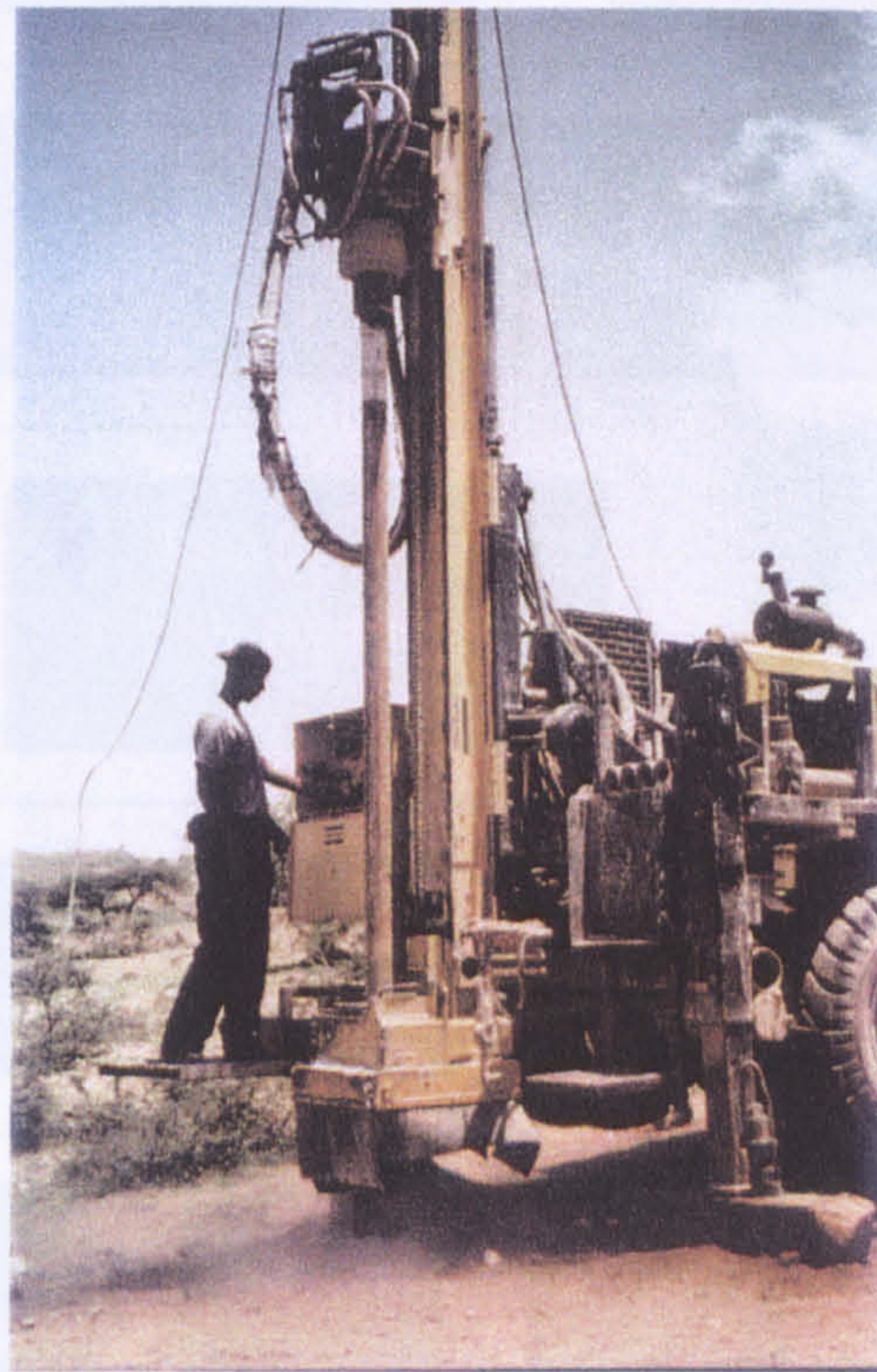
Figure 6.4 Drilling Rig at Kollo Tembien
