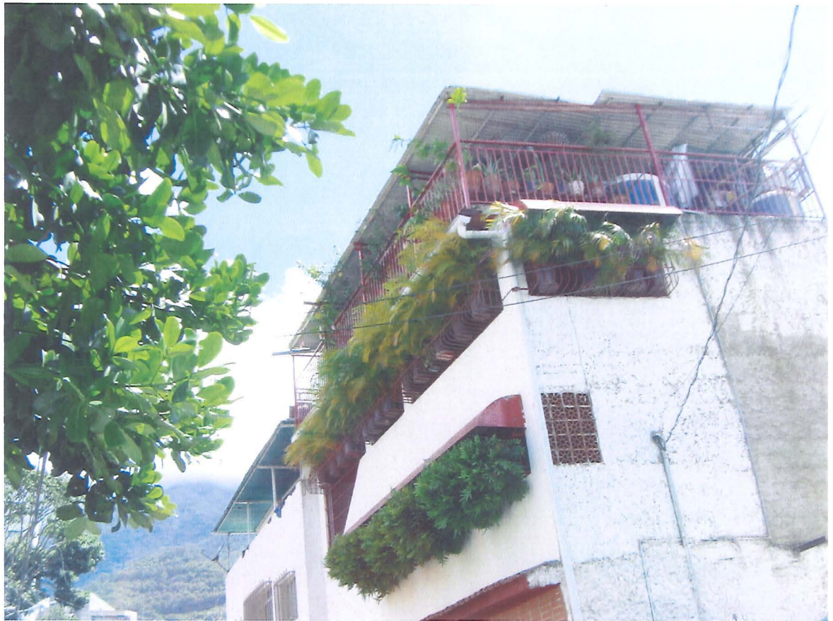
Figure 6.30 - Vertical gardens: Roof patio and plants in windows. Callejon Farfan.
