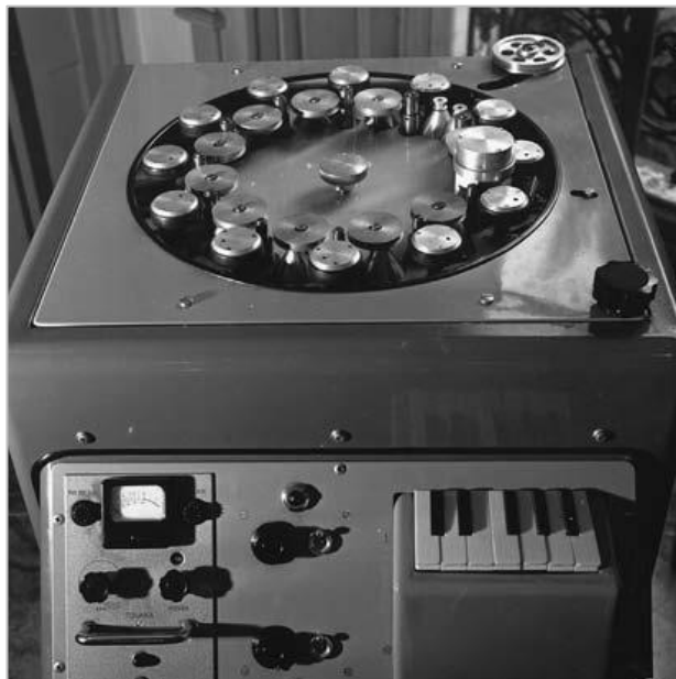
Figure 23: Morphophone with ten audio heads, GRM 1961.
