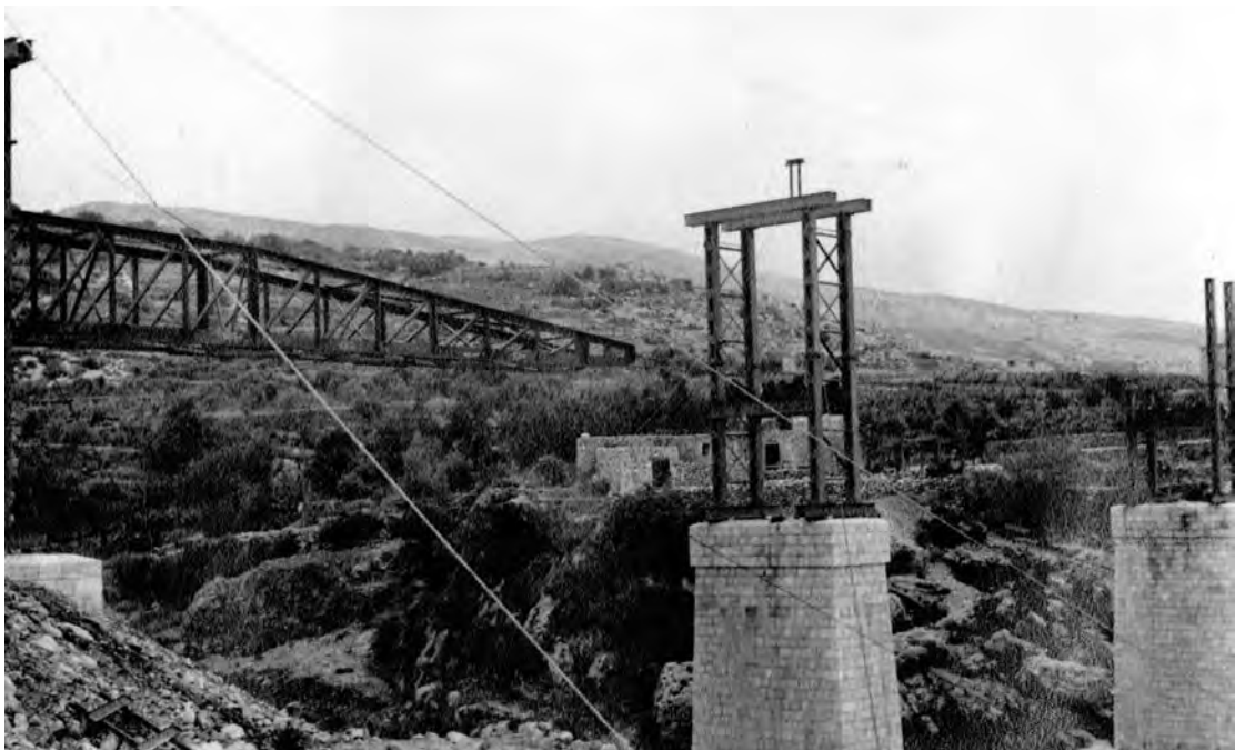
Figure 25: Post-war development of Lebanon's railway. This is the bridge landing over the river in Beirut for the Beirut-Tripoli Railway, 1944. Located at the Middle Eastern Centre Archive.
