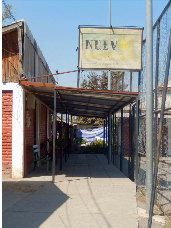
Image 23 Community centre in Nuevo Amanecer Photograph by the author.
