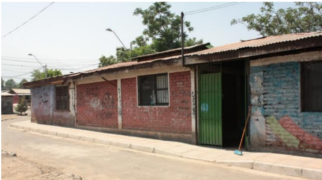
Image 24 Community centre in Nuevo Amanecer Photograph by the author.
