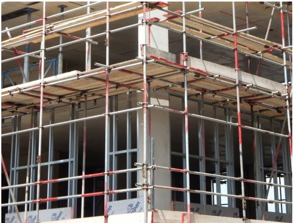
Fig.25 – Construction Site in Deptford (Summer 2014)
