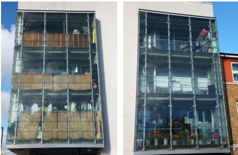
Fig.18 – Consort Road, South Facing Winter Gardens (Spring 2013)
