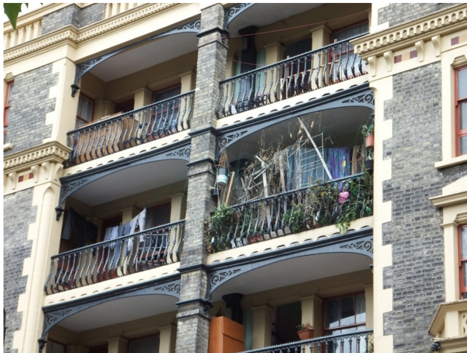
Fig.66 – Leopold Buildings, balcony close ups (May 2014)
