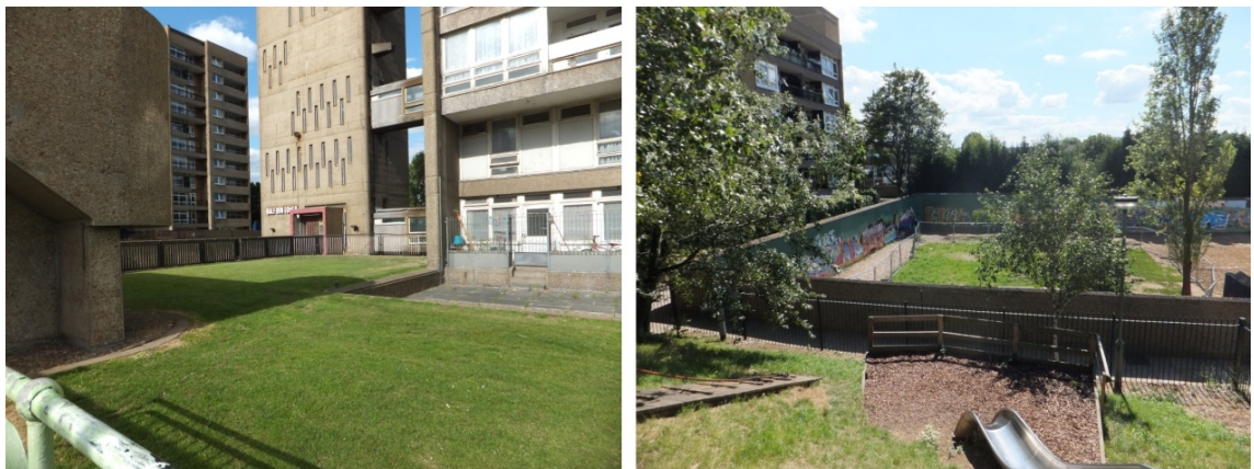
Fig.41 – Landscapes at Balfron Tower (left) and Trellick Tower (right) (Summer 2013)
