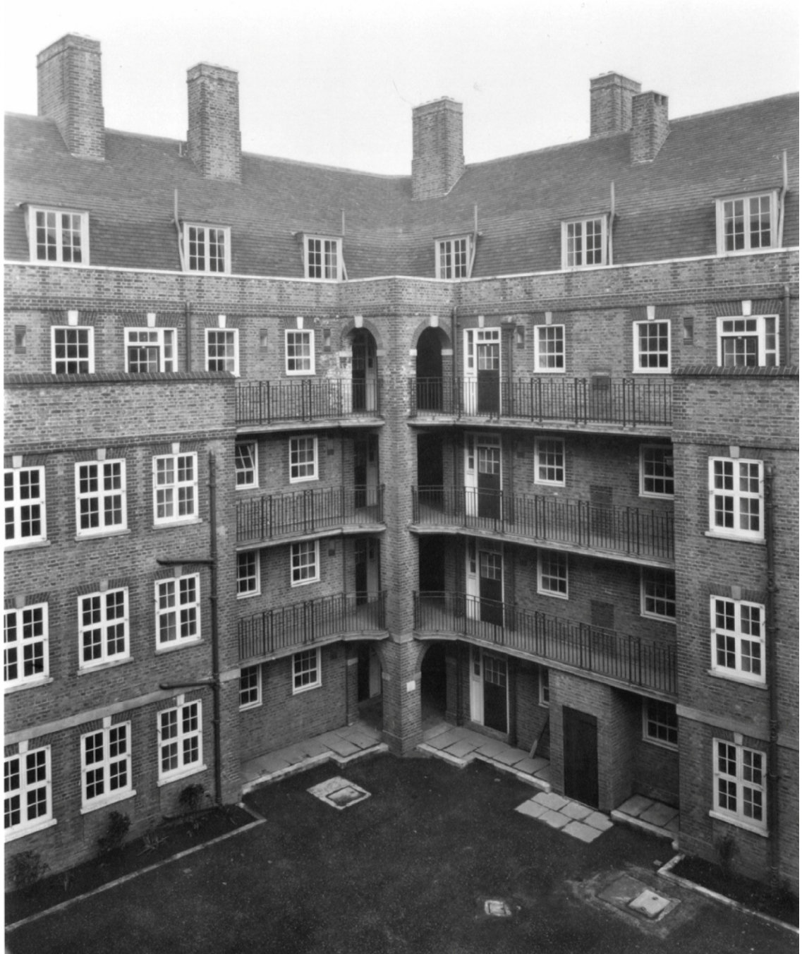
Fig.60 – East Hill Estate, Grassed Courtyards
