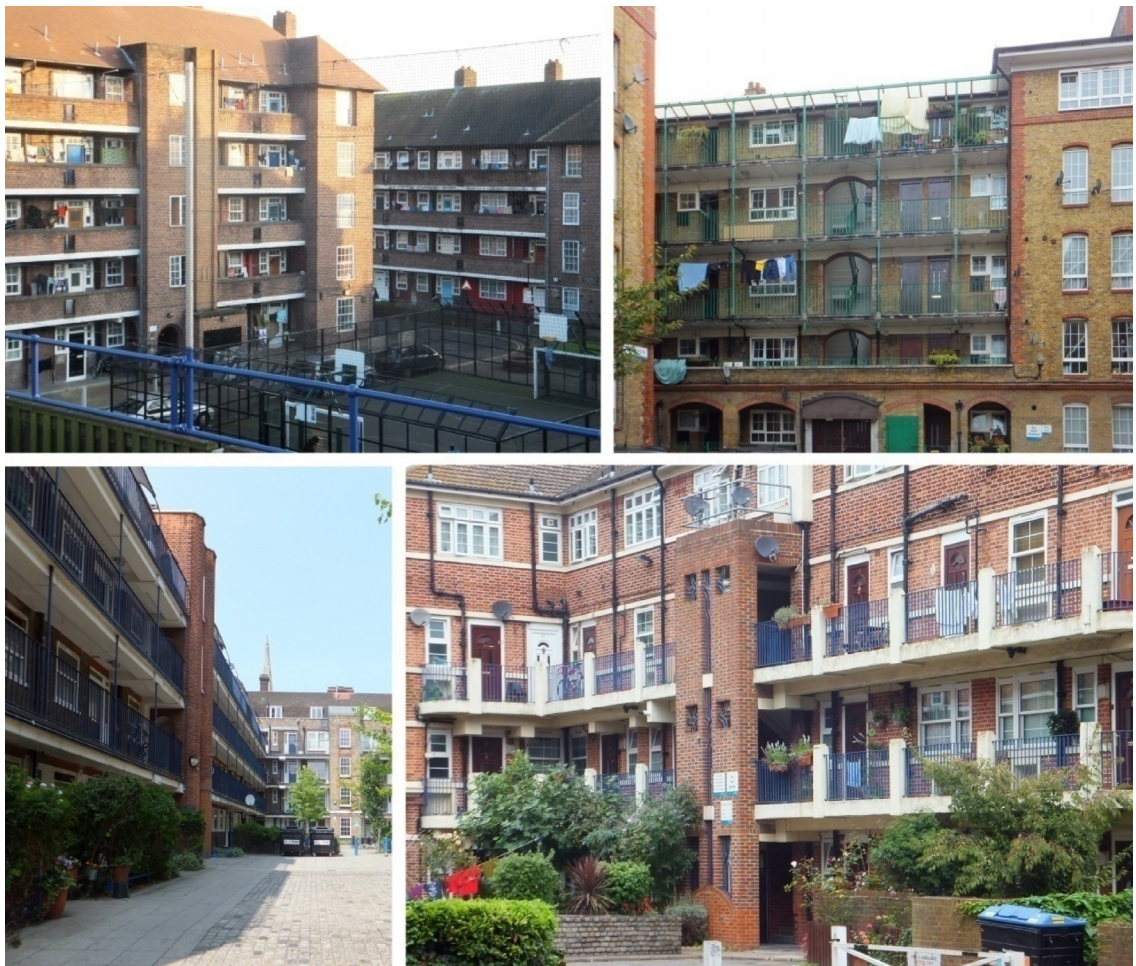
Fig.65 – Balcony Access Council Estates in East and South East London (2013-14)
