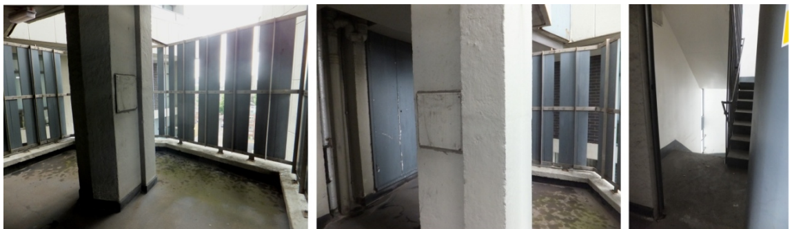
Fig.34 – Keeling House, laundry spaces and stairs (Summer 2013)
