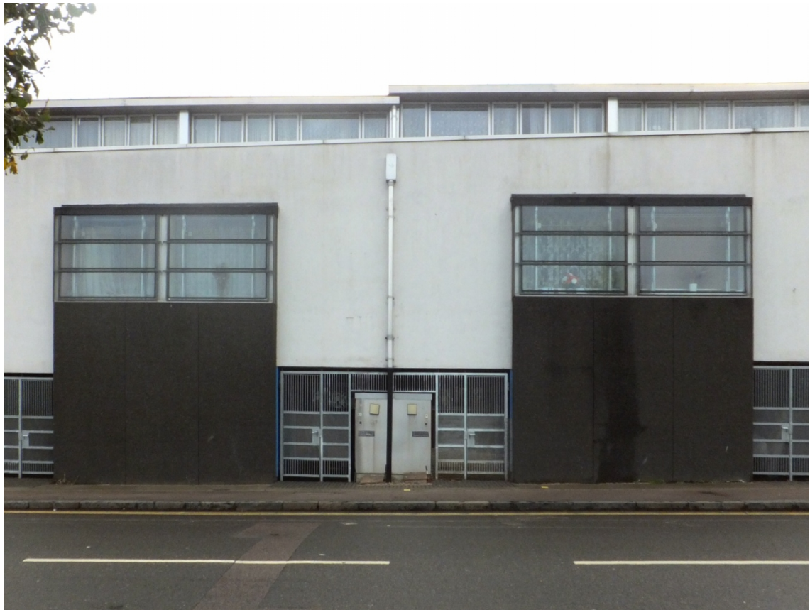
Fig.21 – Twin House Fronts at Consort Road (September 2014)
