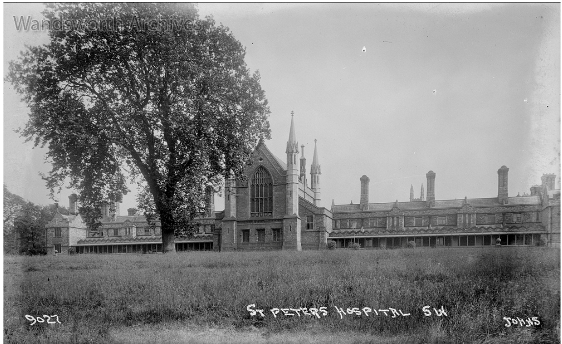
Fig.81 – Back of St Peter's Hospital
