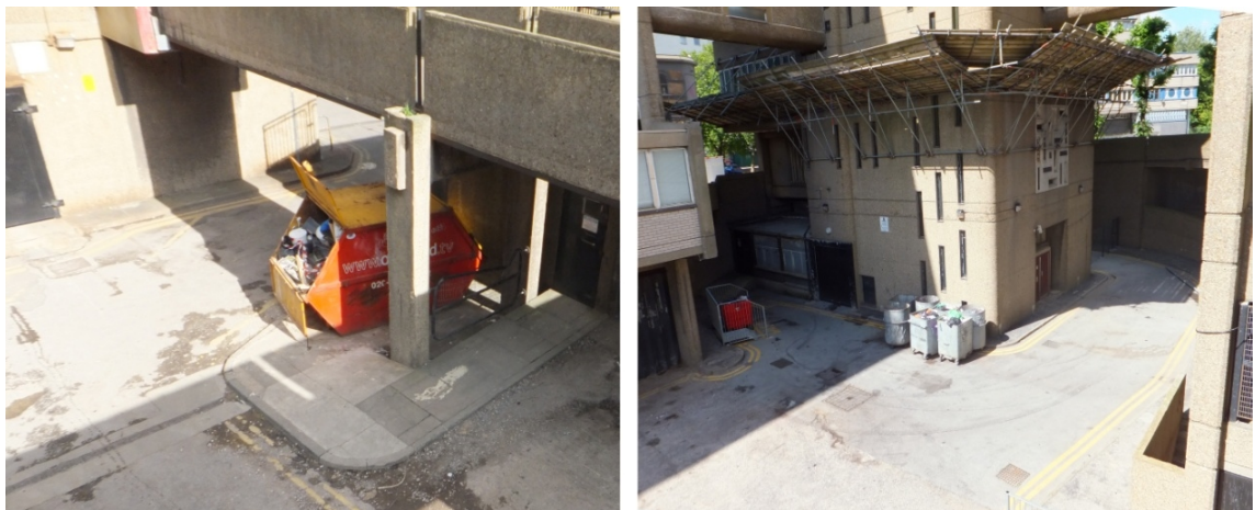
Fig.39 – Base of Balfron Tower core (left) and of Trellick Tower core (right) (Summer 2013)
