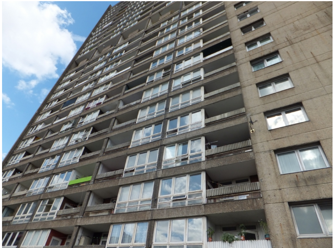
Fig.46 – Balfron Tower, balcony (summer 2013)
