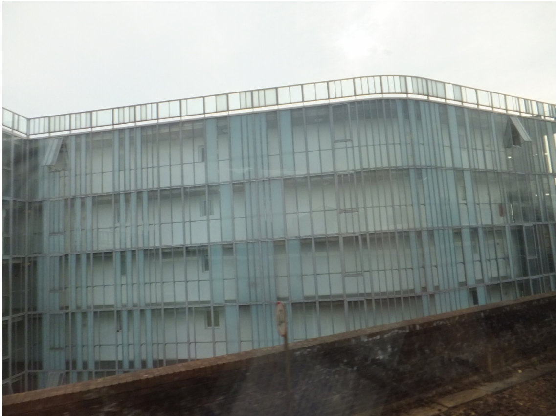
Fig.16 – Consort Road Access Balconies, photograph taken from train (Spring 2012)
