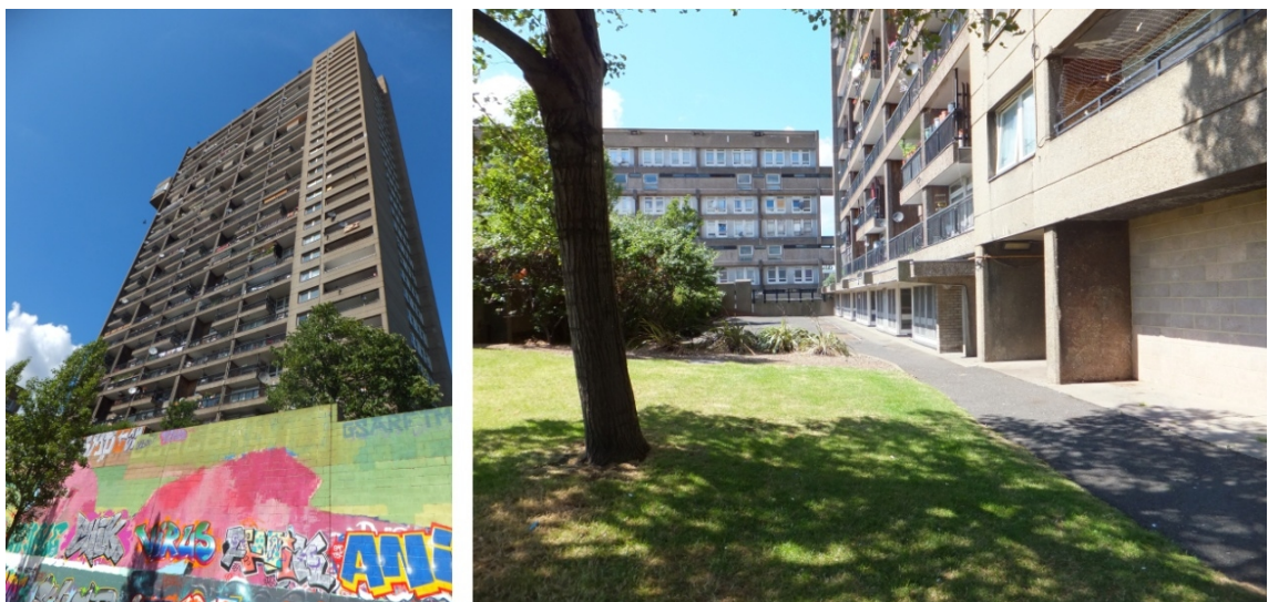
Fig.42 – Trellick Tower, site of former care home, from lower and upper levels (Summer 2013)
