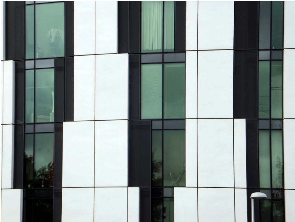
Fig.11 – Exterior of ventilation panels (Winter 2014)
