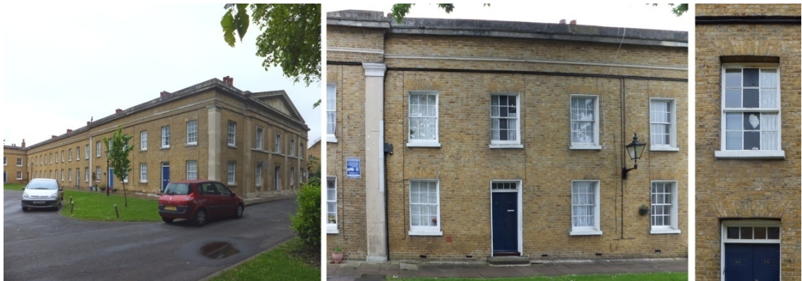
Fig.89 – Caroline Gardens, front of U Shaped building and Window Detail (March 2013)
