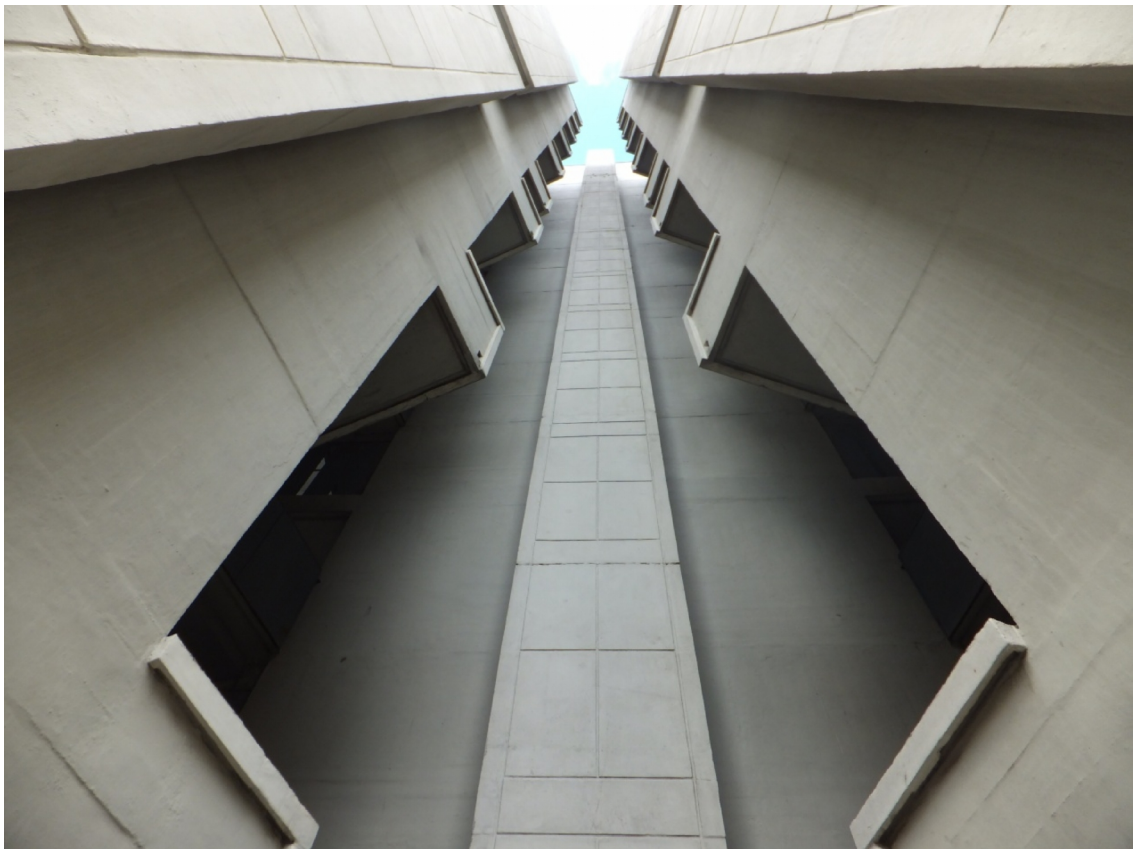
Fig.35 – Keeling House, 'back' view between the two south wings (Summer 2013)
