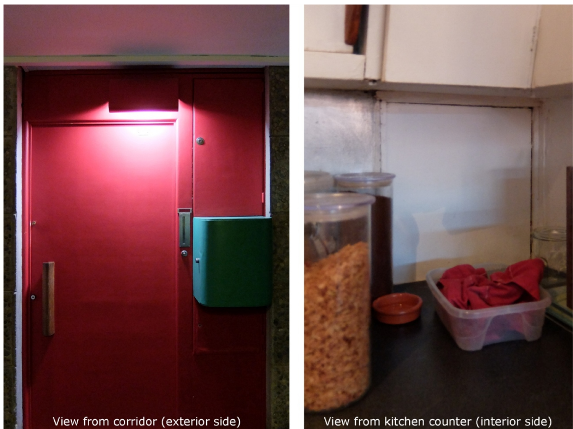
Fig.56 – Delivery boxes at Le Corbusier's Unité d'Habitation, Marseilles, 1952
