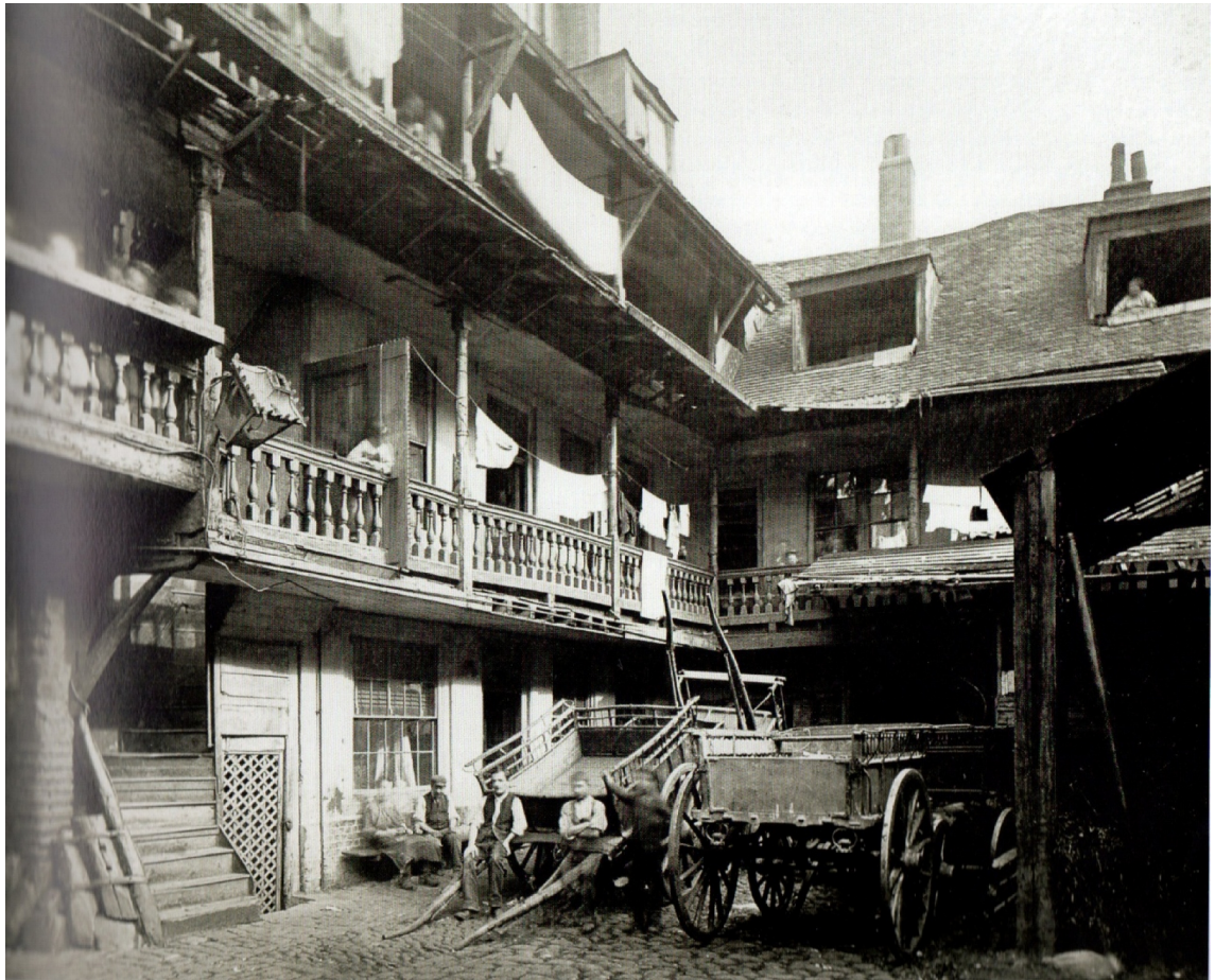
Fig.73 – Oxford Arms, Warwick Lane, 1875
