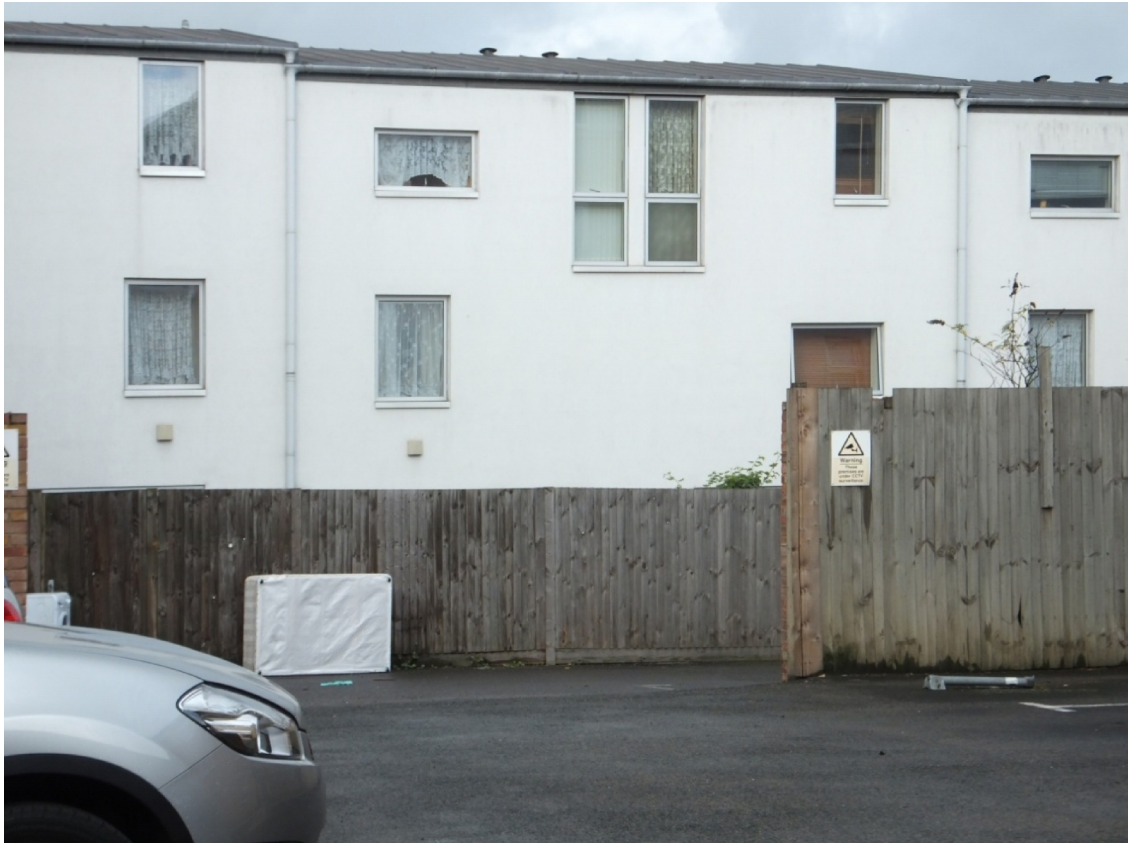
Fig.22 – Back of Terraced Houses at Consort Road (September 2015)
