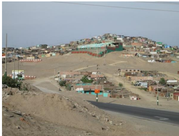
3.6 The green gated building is a public school
