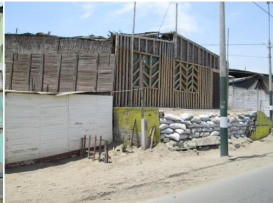
3.15 Sand-bags are also used to hold the houses up.
