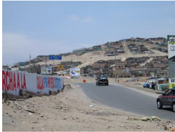
1.2 Road ascending from Ventanilla to Pachacutec
