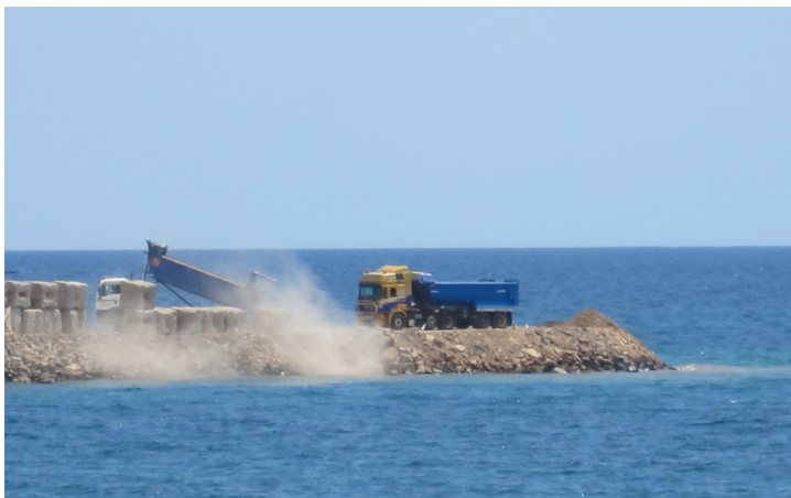
5: Edge of Granadilla port under construction. Tenerife, April 2013.
