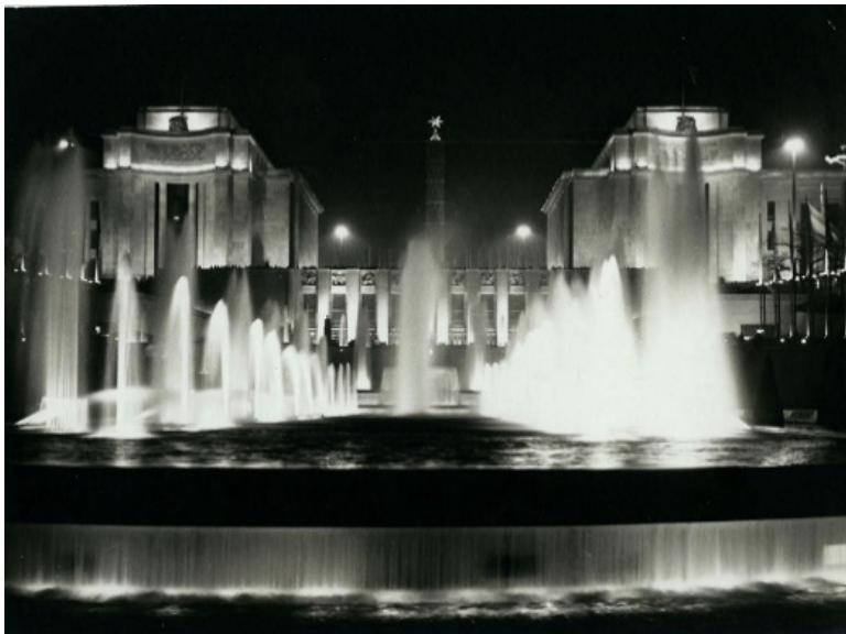
Figure 2. The view of the Palais de Chaillot by night, 1937. The column behind, with the star on the top, was named the Peace Column (it does not exist anymore). By permission of the Bureau International des Expositions.
