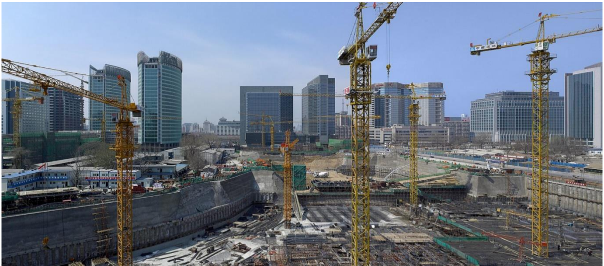
Figure 12: The Beijing Financial Street Centre-Piece Under Construction 41
