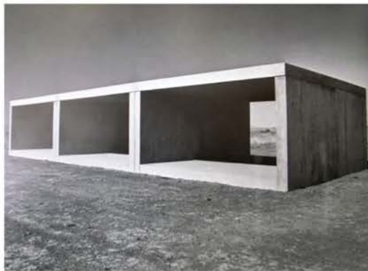
fig.12 Concrete work in three units
