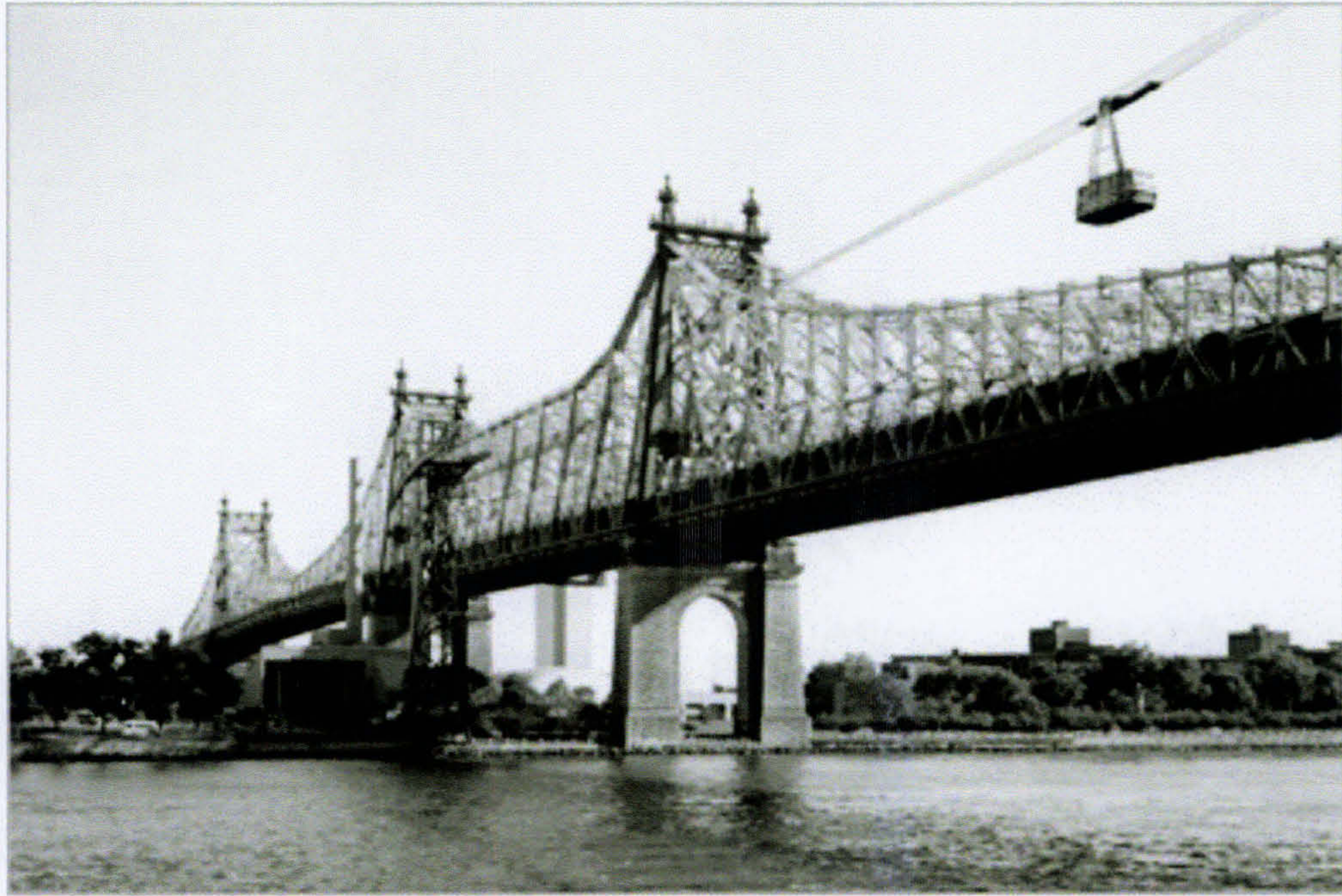
Illustration no. 7, Queensboro Bridge (Douglas Levere, Photographer)
